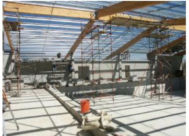
Inside view of lane pool and structural block walls
