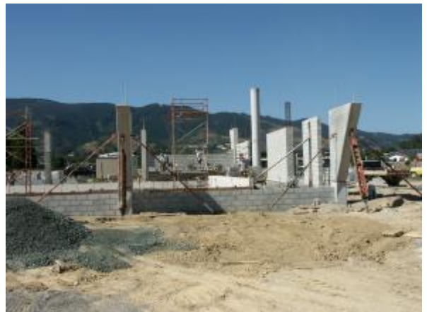
Outside view of lane pool, showing some foundation blockwork.
