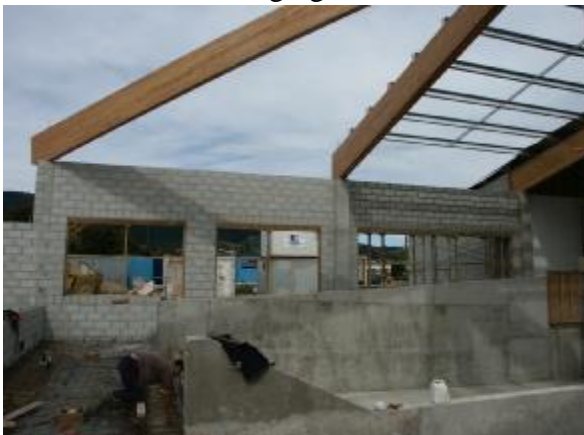
Load bearing blockwork supporting roof above hydro therapy pool
