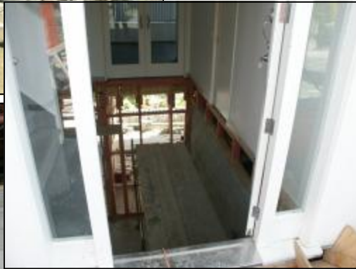
This is the front door after excavation and retaining walls erected
